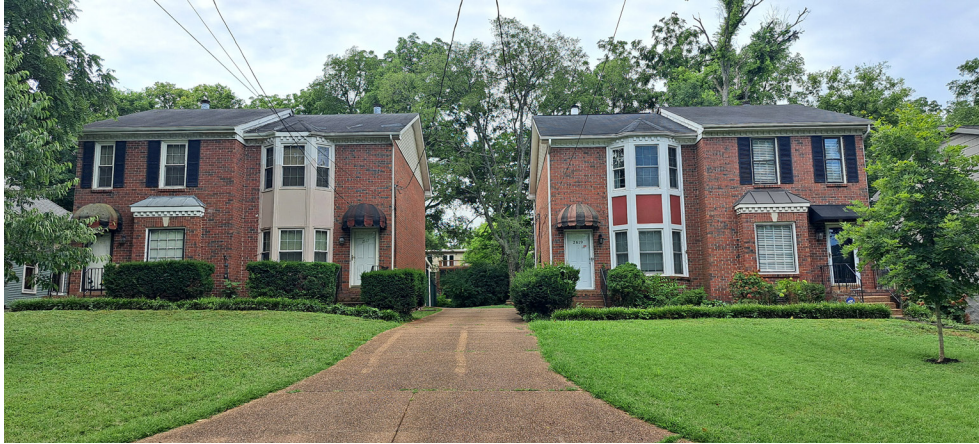
FIGURE 11. Two zero-lot-line duplexes on Westwood Avenue, Hillsboro–West End, infilled in 1985
