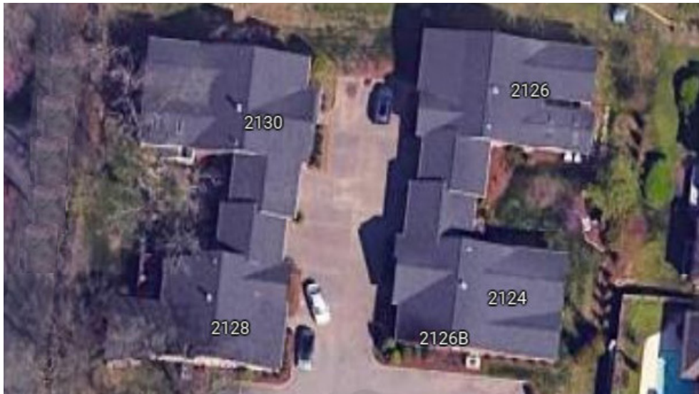
FIGURE 17. Example of two-on-one housing, early 2000s
