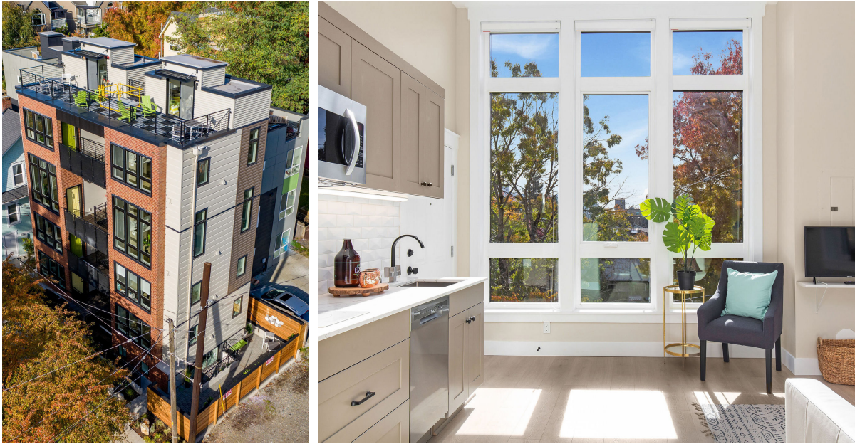
Left: Jansen Court. Right: Jansen Court, interior. Photographs courtesy of CAST architecture.
