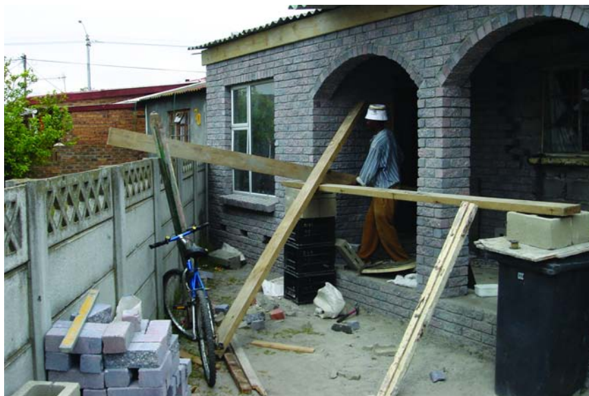
Mrs. Mokhale's front addition, a verandah, in Langa
