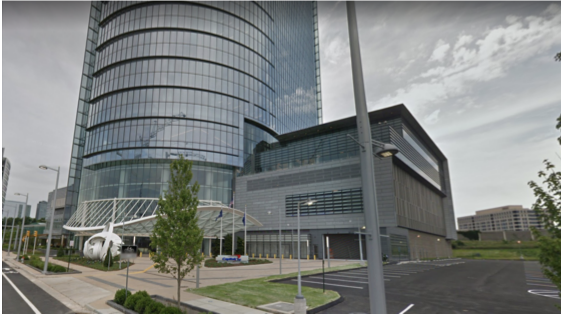
Figure 9. Buildings at Capital One Site
