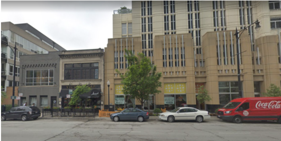
Figure 7. Michigan Avenue in Chicago, Illinois
